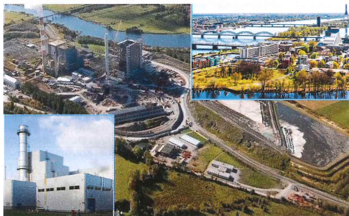
TPP2, one of two 400 MW CC CHP units at the site in Riga
